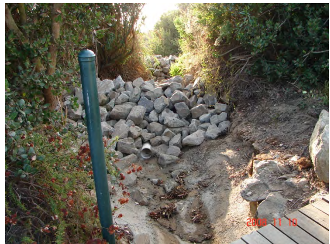
Figure 3: On-site drainage immediately after installation of rip rap (November 10, 2008)
