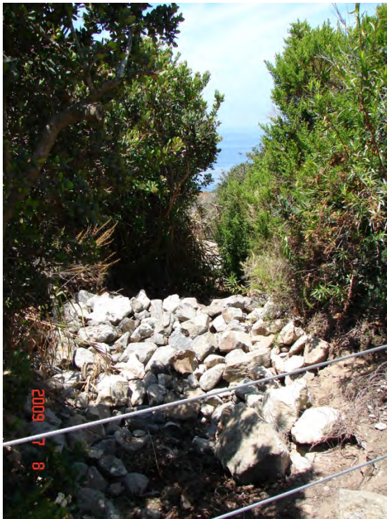
Figure 4: On-site drainage 9 months after installation of rip rap (July 8, 2009)
