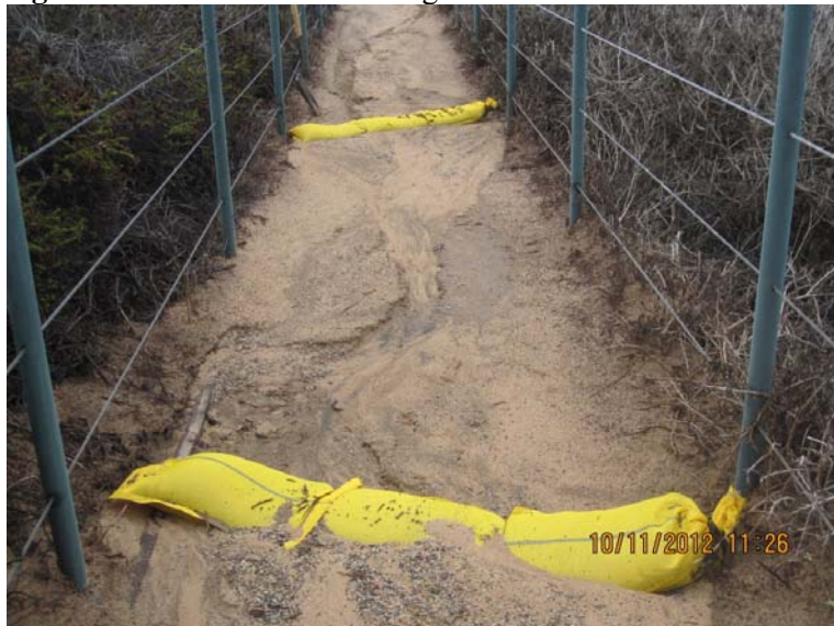
Figure 1: Monofilament Sandbags and Trail Base Erosion
