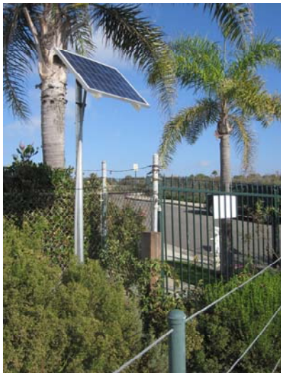
Figure 16: Solar Panel for Gate Lock
