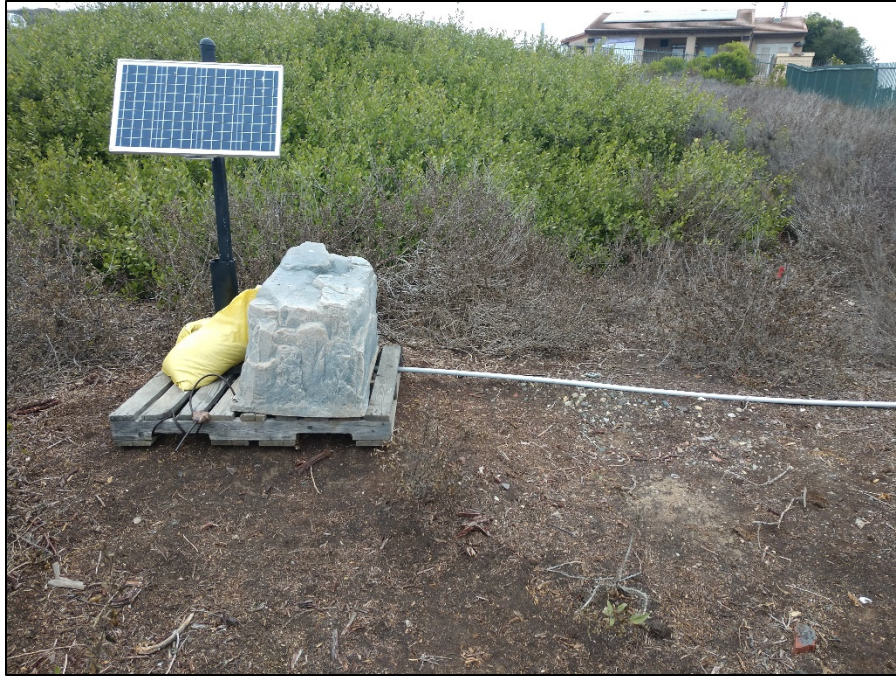
Figure 1. Solar panel and battery at Scenic Gate. The solar panel serves as a reliable power source for the magnetic lock and emergency release mechanism, allowing for safe controlled public access onto CNLM's trail. Photo taken 07/12/2021.
