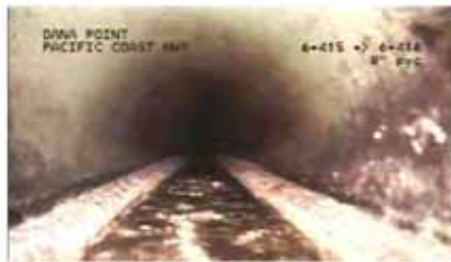
Grease Floating in Sewer Line
