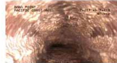
Grease Build Up In Sewer Line
