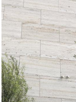
24 STONE VENEER AT STREET LEVEL – TYPE T.B.D. LIGHT BUFF COLOR WITH ARTICULATED JOINTS
