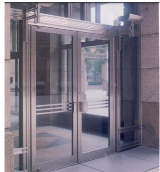
4 METAL STOREFRONT SYSTEMS WITH TRANSOMES AND SPECIALTY DOORS BRONZE ALUMINIUM OR STEEL (T.B.D.)
