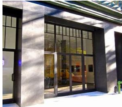
4 METAL STOREFRONT SYSTEMS WITH TRANSOMES AND SPECIALTY DOORS BRONZE ALUMINIUM OR STEEL (T.B.D.)
