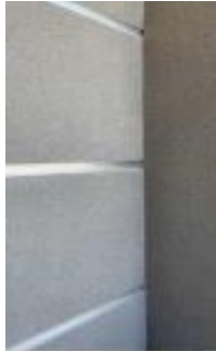
1 LIGHT SAND FINISH STUCCO – ARTICULATED REGLET AND EXPANSION JOINTS WHITE STUCCO AND ALUMINIUM FINISH JOINTS
