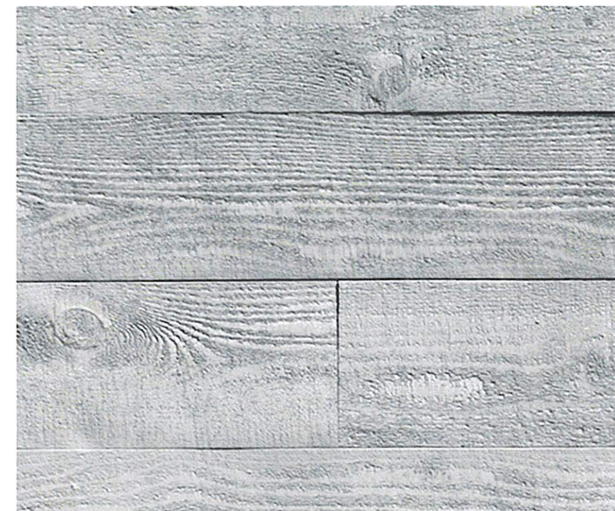
CONCRETE 2 - BOARD FORM
