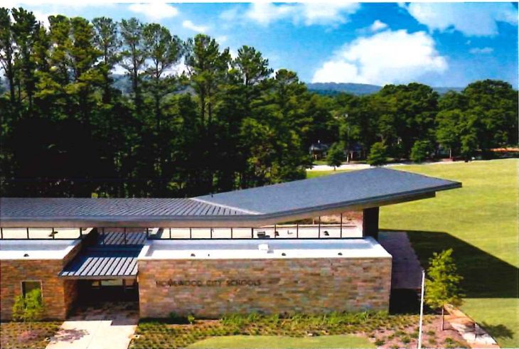
Standing Seam Metal Roofing • Manufacture: Pac-Clad • Class "A" Metal Roof • Color: Gray or Midnight Bronze "Black"
