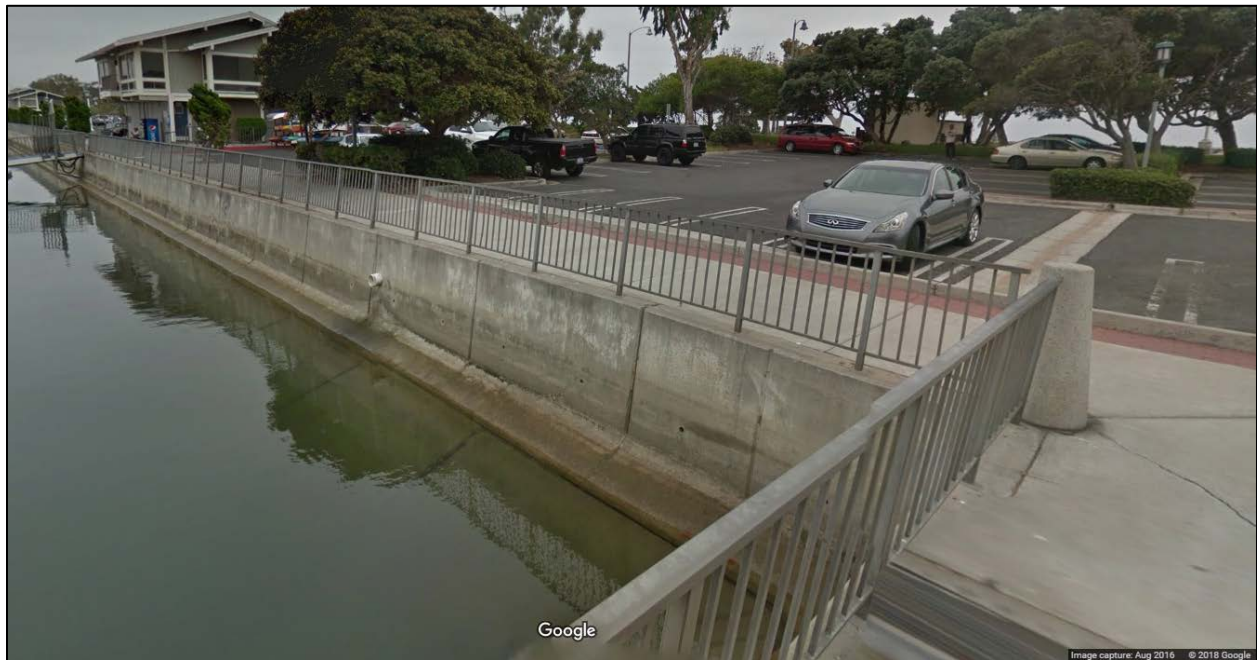
Figure 7-4: Photo of Typical Edge Condition for Dana Point Marina: Concrete Bulkhead with Rail Fencing (Google Streetview 2016)
