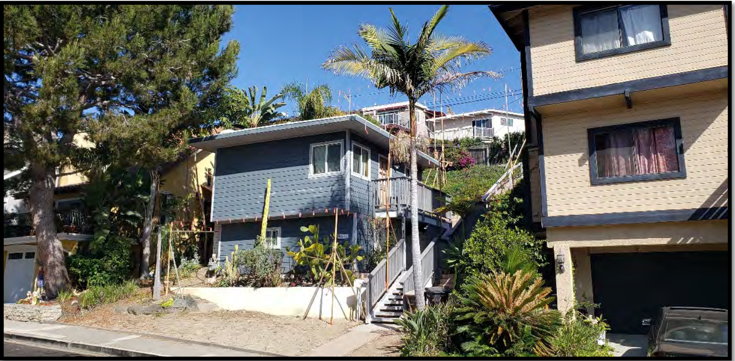
VIEW OF EXISTING DWELLING FROM ROBLES DRIVE
