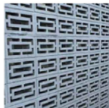
BREEZE BLOCK MASONRY UNITS MFR: ORCO BLOCK & HARDSCAPE COLOR: DUNN EDWARDS - FLINSTONE (DE6221) LOCATION: ENTRY COURTYARD WALL
