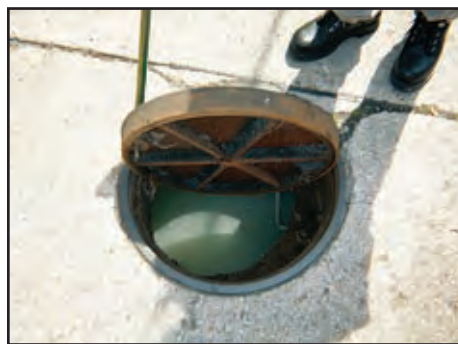
Figure 55: Manhole observation (left) indicates a sewage discharge. Source is identified at an adjacent sewer manhole that overflowed into the storm drain system (right).
