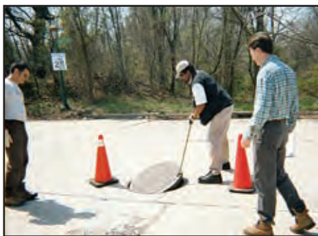
Figure 55: Manhole observation (left) indicates a sewage discharge. Source is identified at an adjacent sewer manhole that overflowed into the storm drain system (right).
