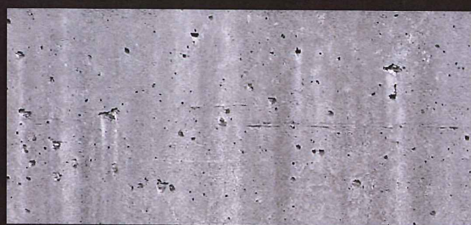
Poured in Place Concrete
