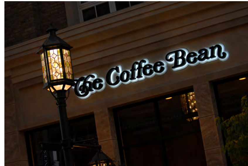
Strong LED backlighting of signage brings attention to retail spaces.
