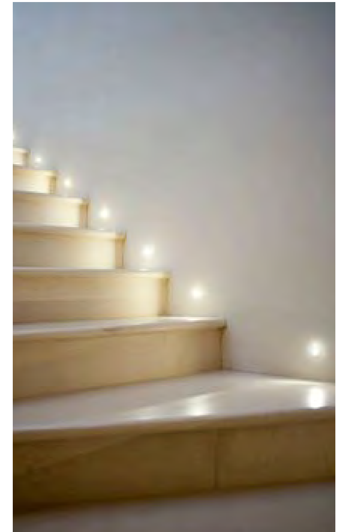
Stemplights mounted on the interior walls of the stairwells evenly washes the steps providing safe and comfortable illumination.
