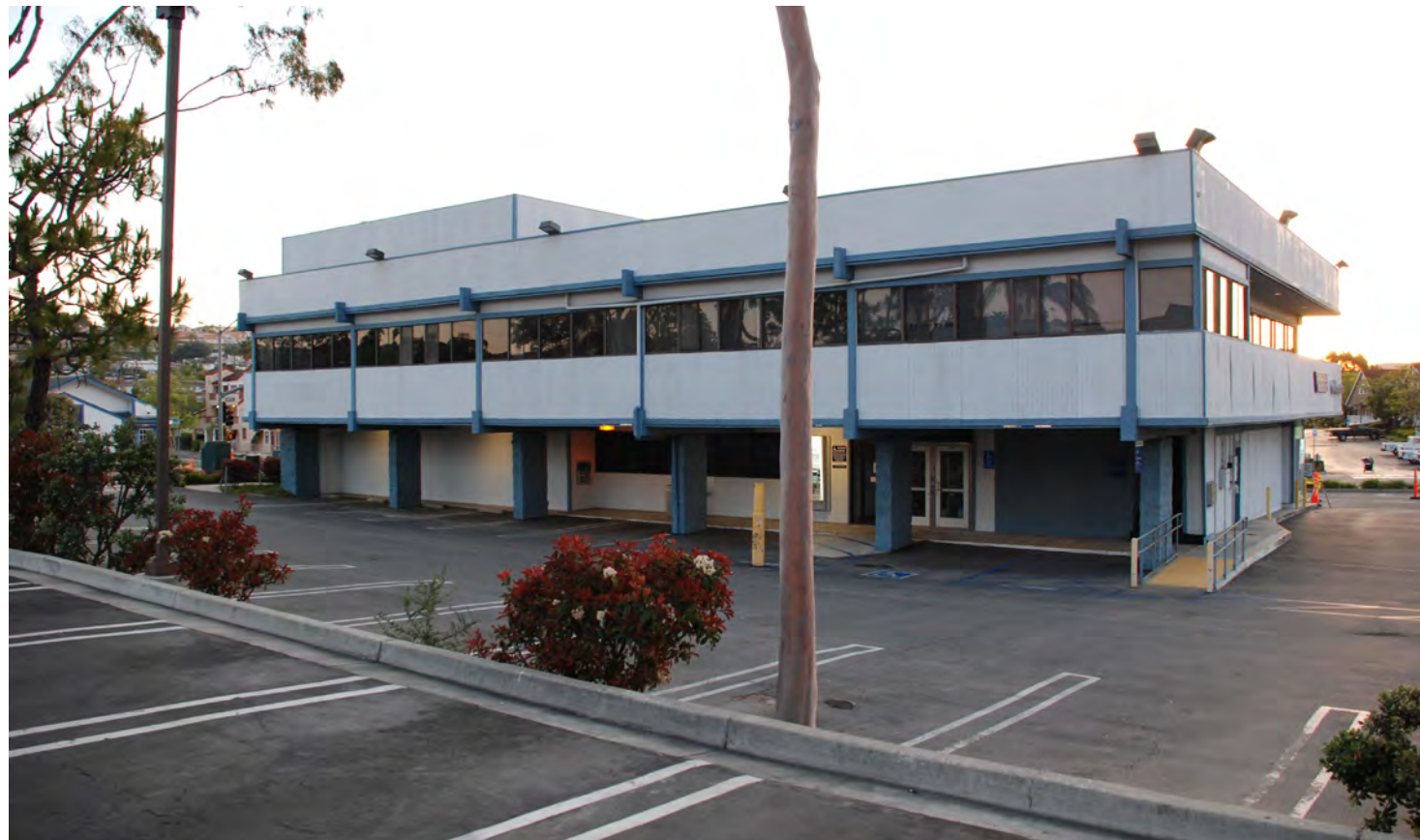
NE view toward site
