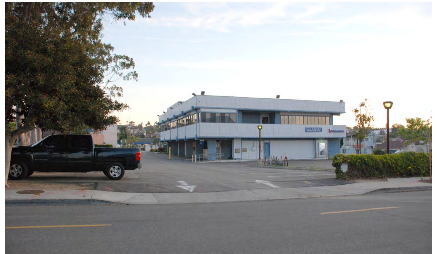
NE view toward site
